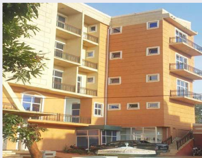
Financed Project-Bamboo Paradise Hotel-Assosa
